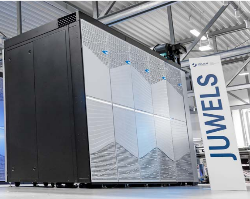
JUWELS supercomputer in the computer hall of the Jülich Supercomputing Centre
