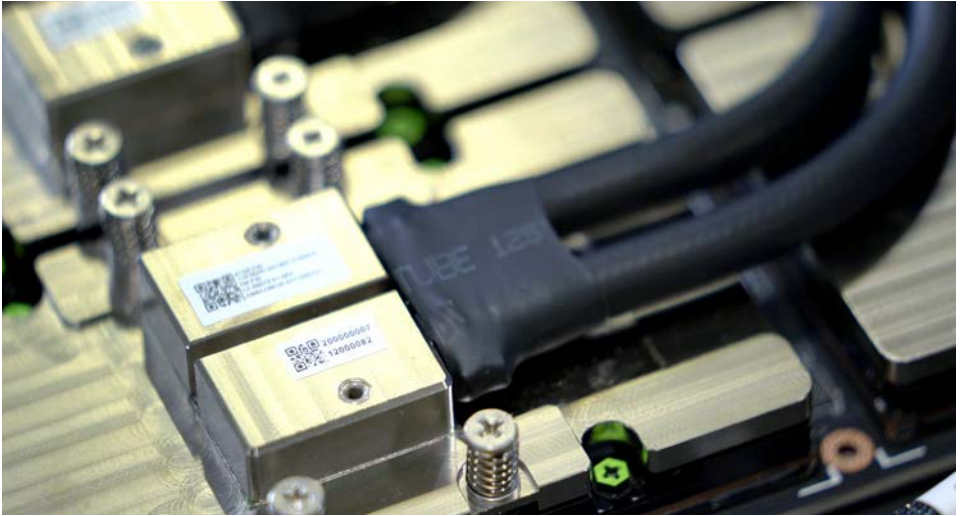
Water cooling in the JUWELS supercomputer
